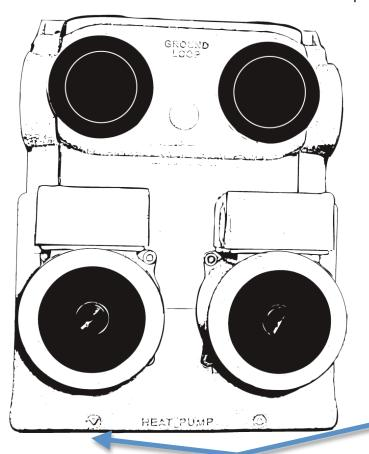
Looking at the bottom connection, left hand side. If installed properly, the pump impeller should be visible.
